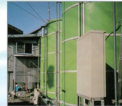
FRP Treatment Tank
